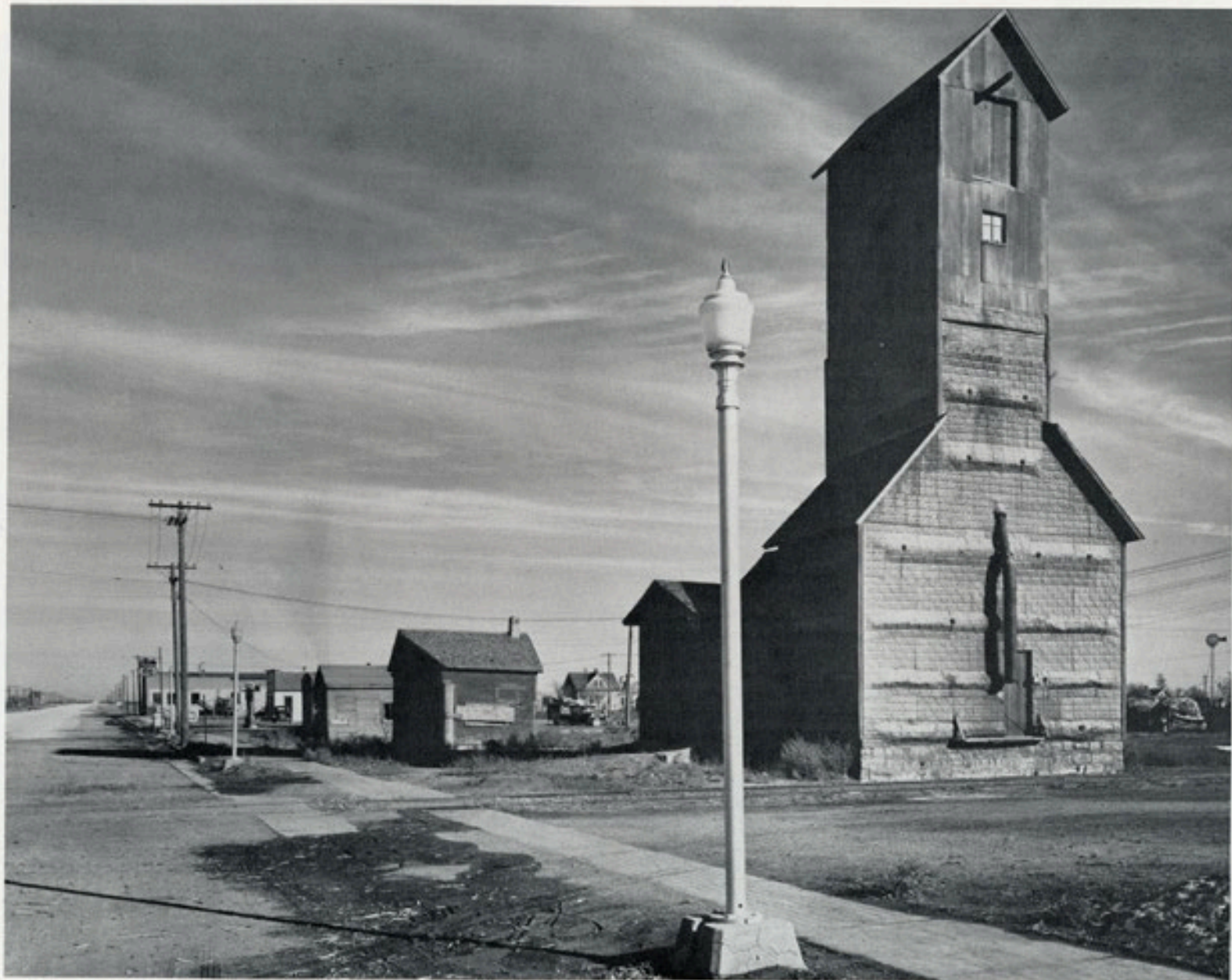
Grain Elevator and Lamp Post, Nebraska, 1940
